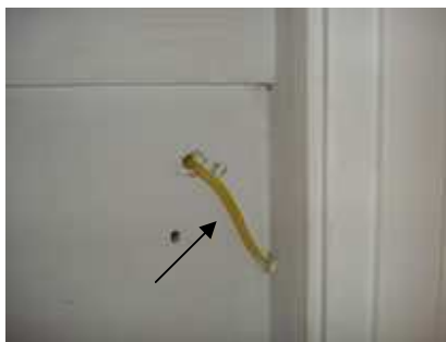
Unprotected Wiring
