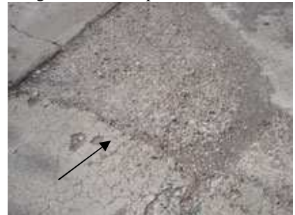
Driveway Deterioration
