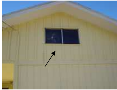
Replace Window With Gable Vent
